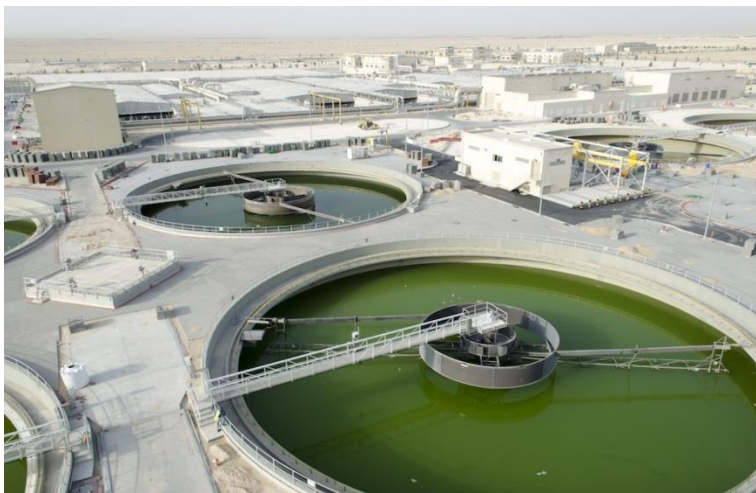
Fig.1. Sewage treatment plant
