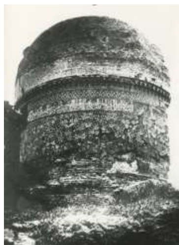
Figure 3: The condition of the dome of Suyunch Khan mausoleum before the earthquake. Photo by D. Ermakov, archive Glav NPU.
