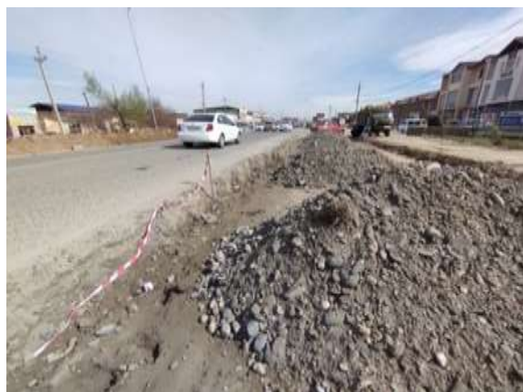
Fig. 1. Nurabad district, road construction "4N 513 Chunkaymish".
